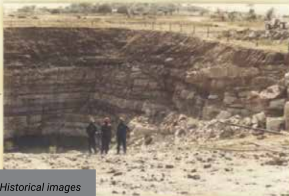
NORTH ADIT - DRILLING IN PROGRESS.
