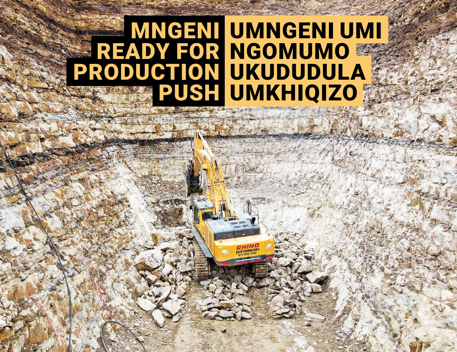
The removal of hard rock at ZAC's new Mngeni Shaft / Kugugulwa amatshe emgodini omusha we-ZAC, uMngeni Shaft
